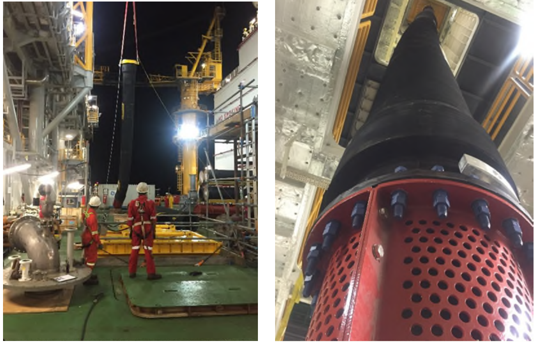
Fig.2-4: Installation of PFLNG1 Seawater Intake Riser
