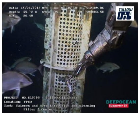
Fig.7-2: Jet Washing of Strainer
